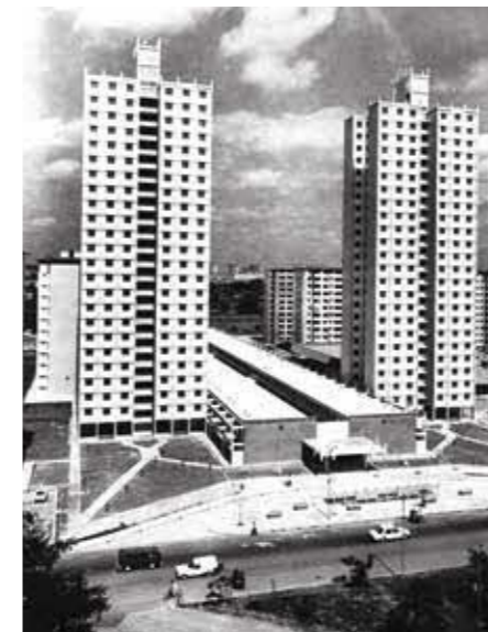
(Left) The first HDB "point blocks" – at 20 or 25 storeys high – were built in the late 1960s. In this photo taken at Bendemeer Road in the 1970s, the "point blocks" tower over the surrounding rectangular "slab blocks". In between the point blocks is a row of low-rise shops. Courtesy of National Archives of Singapore.
